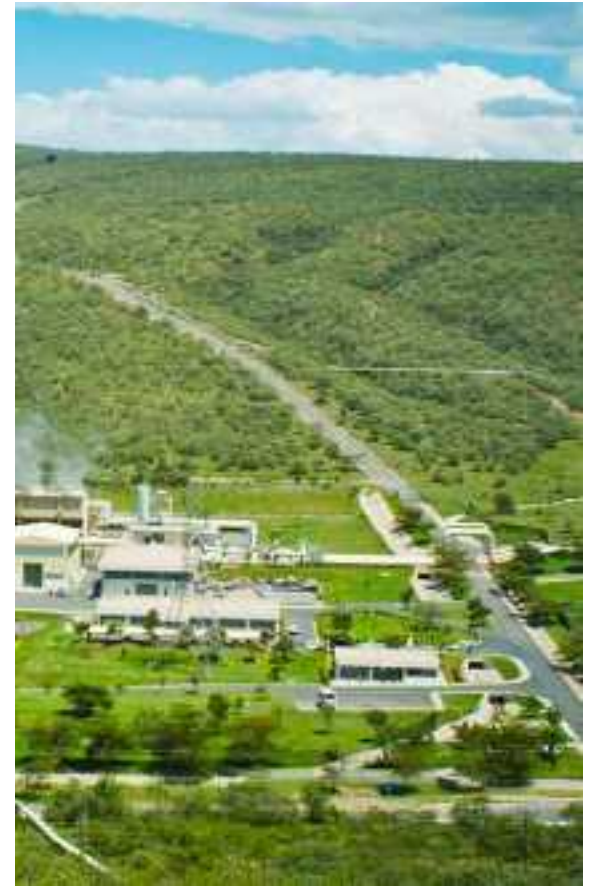
Geothermal underground power plant
